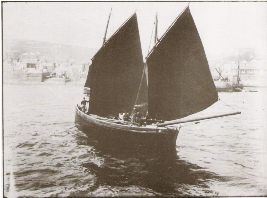
This is the General Havelock, a mackerel boat entering the harbour. It is a square rig boat that is not often seen now. There are two sails the same size but usually the mizzen is smaller.
